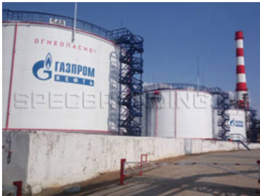
Figure 1 - UKPGiK 500 Tank Farm
